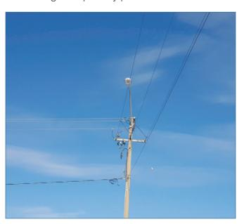
Or here in this double fail where the light in the foreground is too close to the primary cable and the one in the background is mounted on a loose metal extension on a wood pole:
