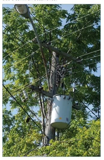
Other safety issues include the utility laying secondary cables across the back of the davit arm when they installed new poles:
